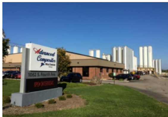
New facility site at Advanced Composites, Inc.
