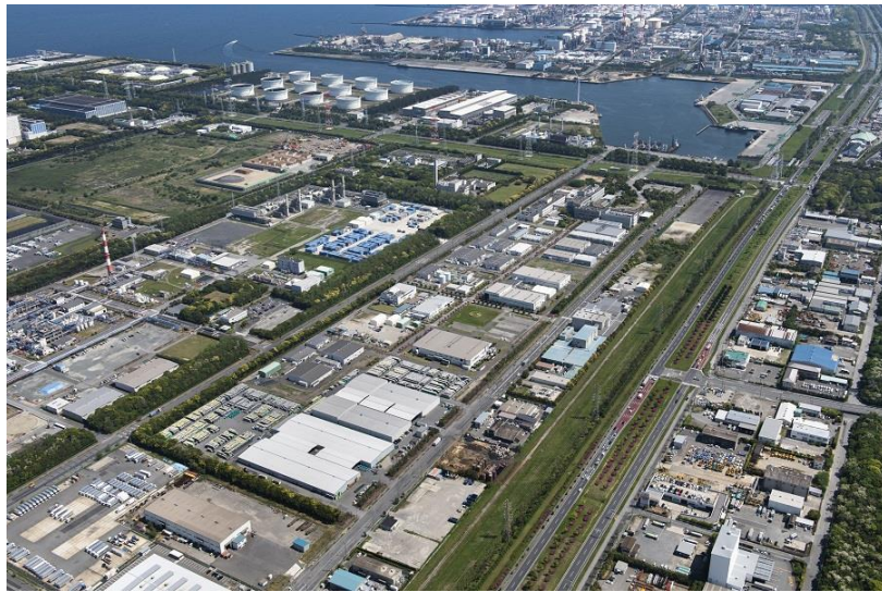
Aerial view of the Sodegaura Center
